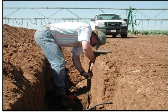
Figure 10. Connecting SDI laterals to manifolds and flush lines at TAES, Halfway, 2006.
